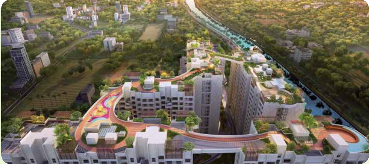
Aerial view of Rooftop Skywalk
